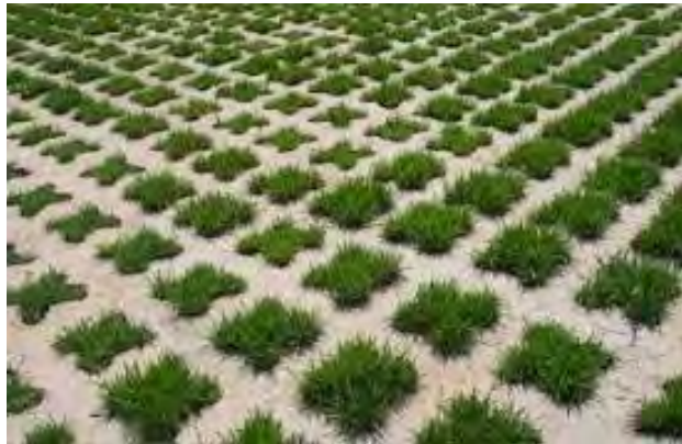
Turning Head & Fire Tender Access Grasscrete
