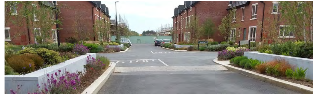
Extensive planting to provide traffic calming in the form of vertical deflection.
