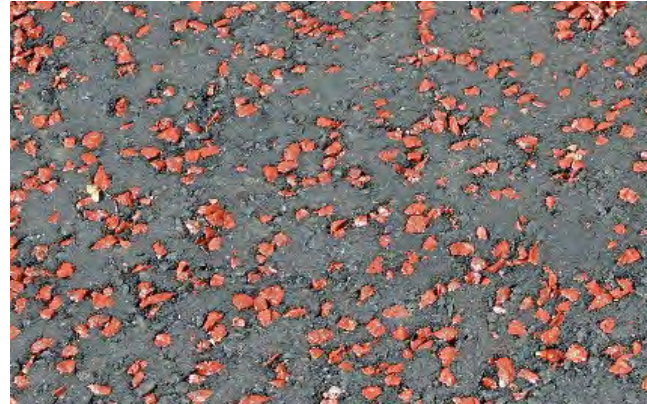
Internal Junctions Tarmac with colour chip
